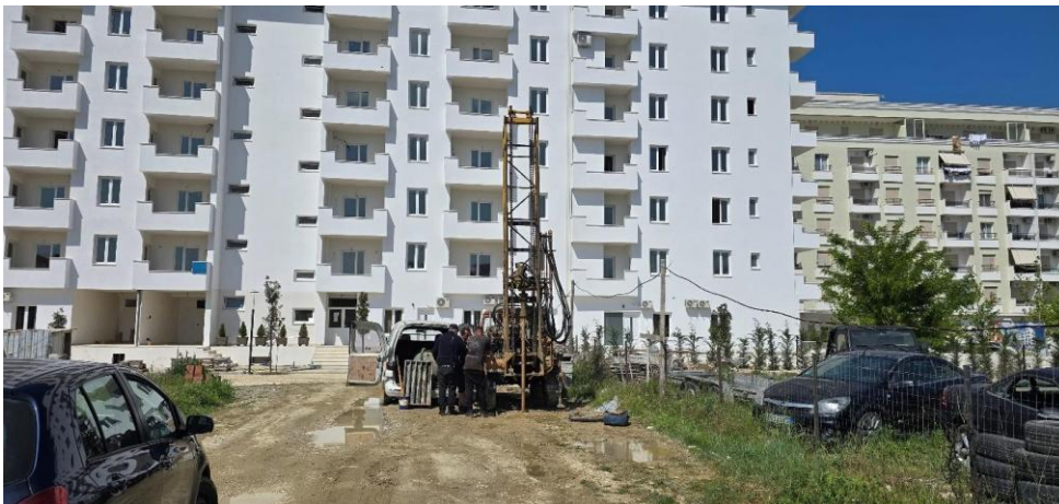
Fig.4 Photo during the drilling of borehole no. 1. Source [6]
