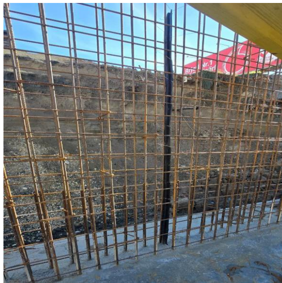
Fig.12 Waterstop for targeted crack stimulation Source: Authors
