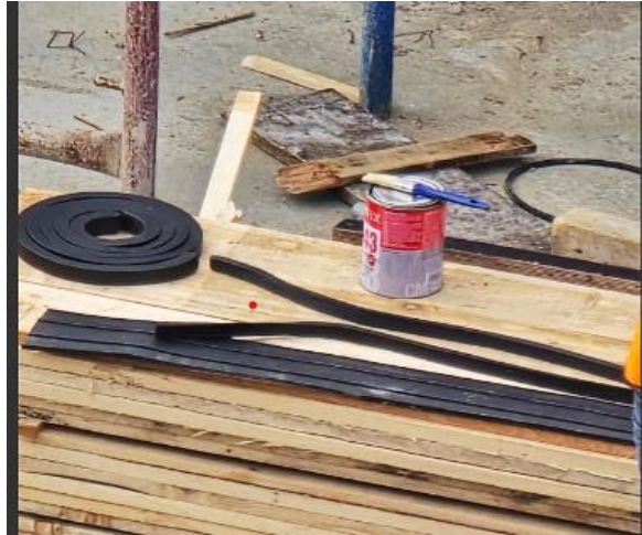
Fig.10 Expansive waterstop 20x25 Source: Authors
