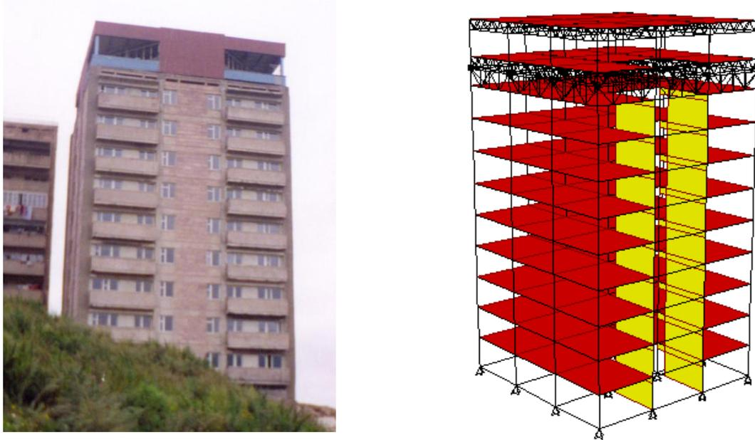
**Figure 1.** General view of the apartment building, the seismic resistance of which has been increased by the method of additional seismic isolated upper floor (proposed by the author of this paper), and the design model of this building
