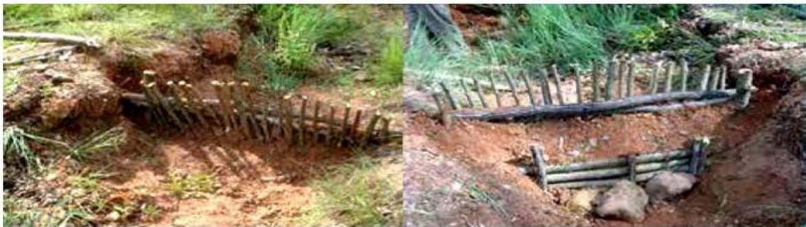
Figure 6: Palisades (Source: Road side Bio-engineering, Site Hand Book, John Howel)
