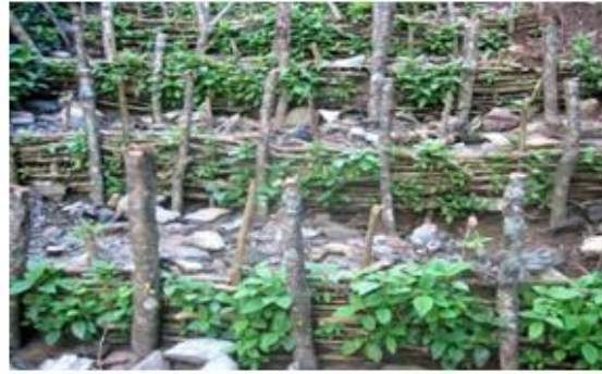
Figure 7: Live Check Dam (Source: Road side Bio-engineering, Site Hand Book, John Howel)
