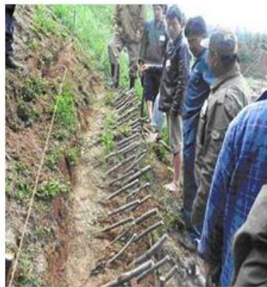
Figure 5: Brush Layering (Source: Road side Bio-engineering , Site Hand Book, John Howel)
